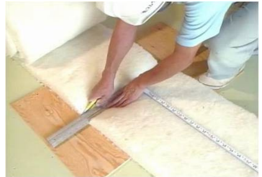
Rams Insulation is easy to cut by using either scissors or tearing the batt across the width.
