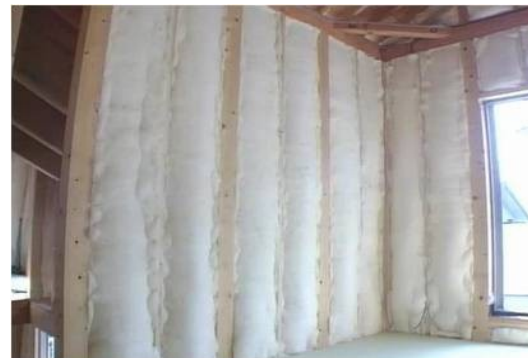
Installing Rams Insulation correctly will save you energy costs through-out the summer and winter months.
