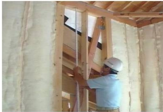
Before installing insulation ensure a qualified electrician has securely fixed electrical wiring to the stud wall or ceiling.
